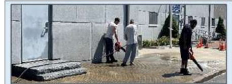
Under the supervision of Hardscape Instructor Dave Collins, participants replaced the large section of brick in front of our Middleton facility
